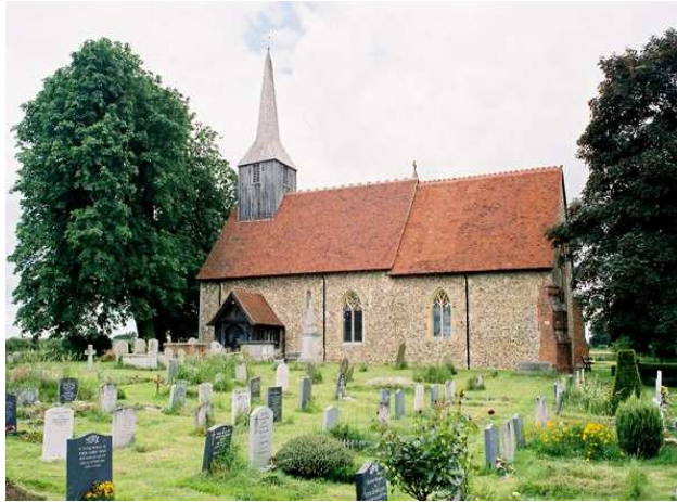
Black Notley church from the south side
